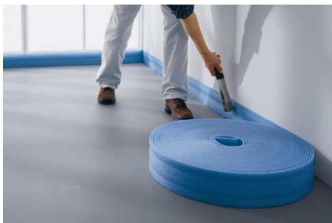
Fig. 1. Installation the damper tape
