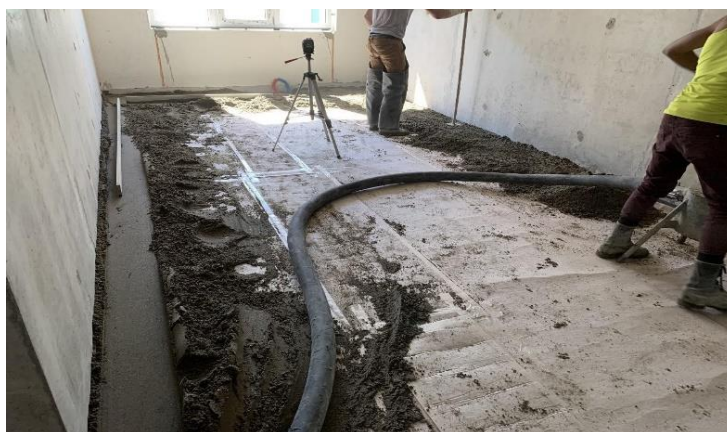
Fig. 4. Installation of a cement-sand screed
