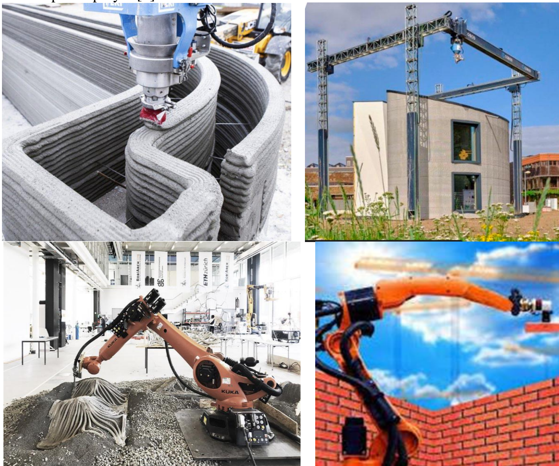
Fig. 1. Examples of modern 3D construction printers and KUKA robots in construction [11]
