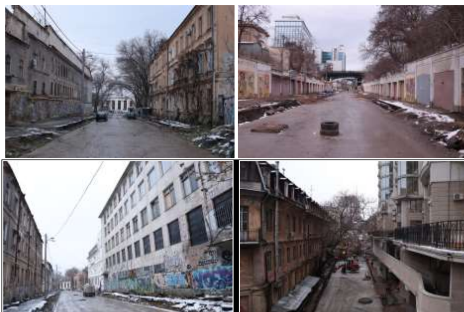
Fig. 5. The technique of reflecting negativity in the construction on Devolanovskiy Descent in Odesa.
