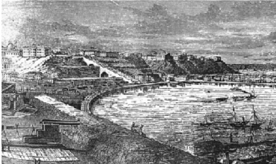
Figure 3. Landscaped slopes of the plateaus with terraces and retaining walls
