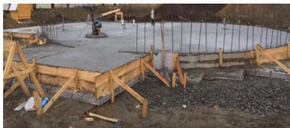
c – setting monolithic slab
