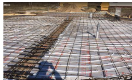
b – reinforcement placement
