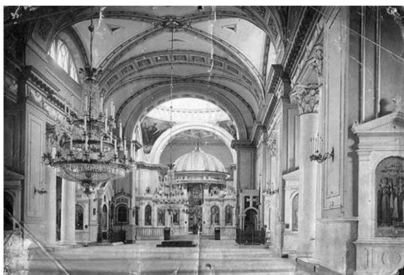
Fig. 11. The interior of the Cathedral after reconstruction in 1900-1903 years. The central nave
