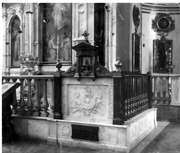
Fig. 10. The interior of the Cathedral after reconstruction in 1900-1903 years. The grave of duke Vorontsov
