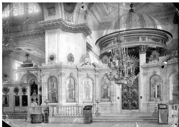
Fig. 9. The interior of the Cathedral after reconstruction in 1900-1903 years. The main altar
