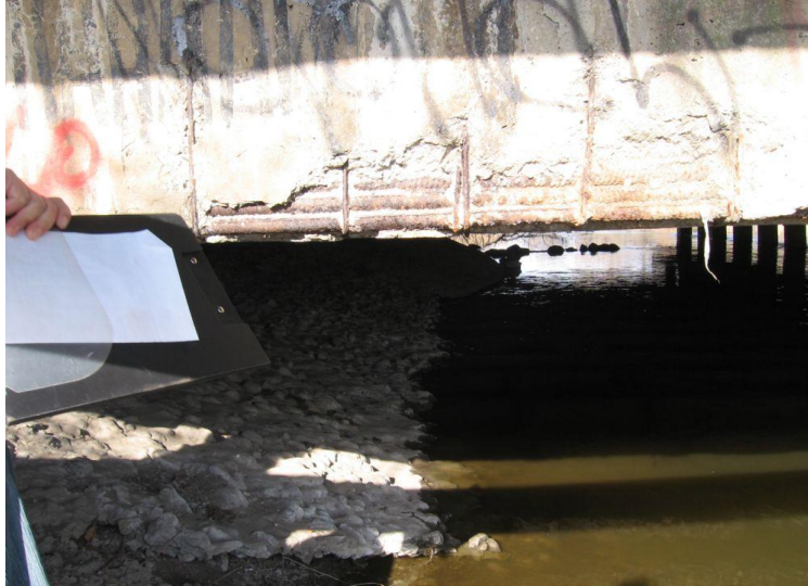
Fig. 1. Concrete spalling, exposed and corroded reinforcement of the bridge deck girders
