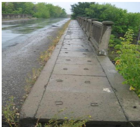
Fig. 3. Partial lack of bridge railing and damages of the road dressing
