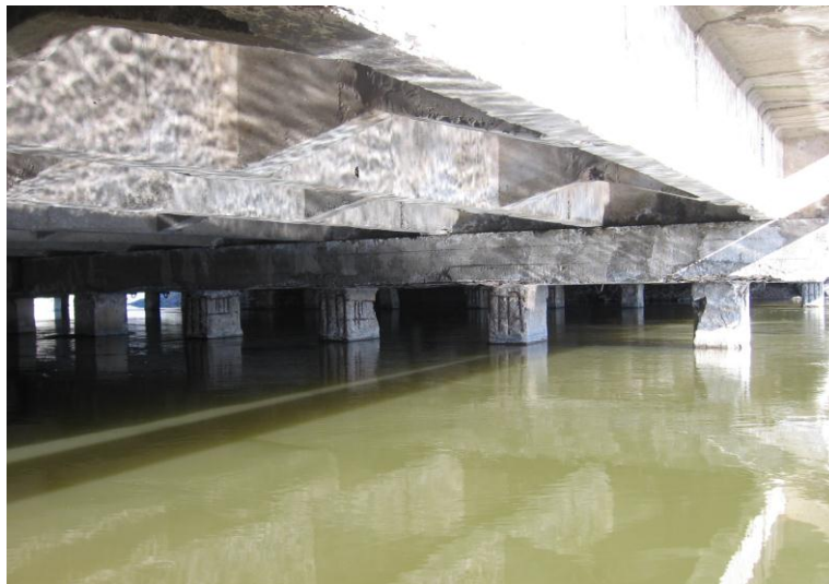
Fig. 2. Concrete spalling, exposed and corroded reinforcement of the bridge piles
