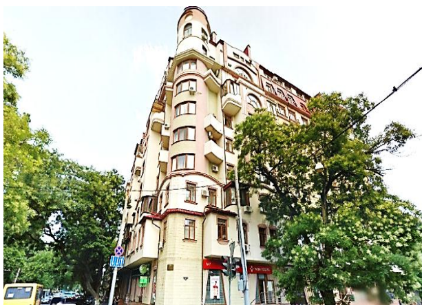
Fig. 1. Reconstruction of a residential building in Odessa – the corner of Polska Street and Devolanovsky Descent
