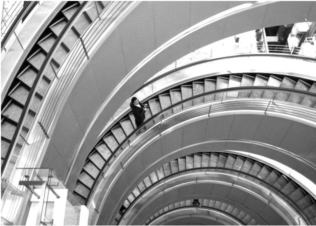
a) The spiral escalator in the department store New World Daimaru. Shanghai. China [4]
