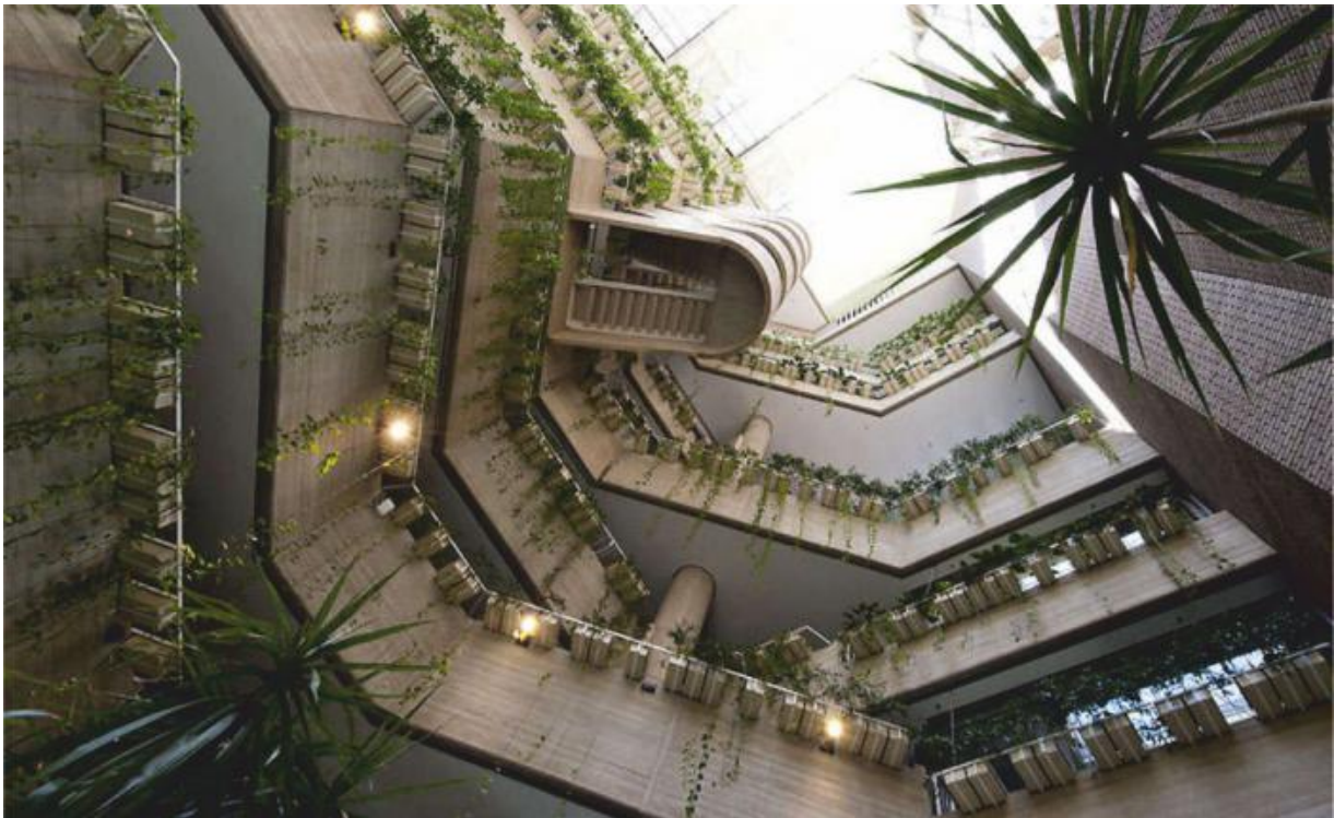
Fig. 1. Atrium in the office building of "Scandinavian Airlines" 1987, Stockholm, architect. N. Thorp
