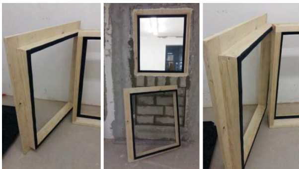
Fig. 1, 2, 3. Experimental installation of sound insulation panels
